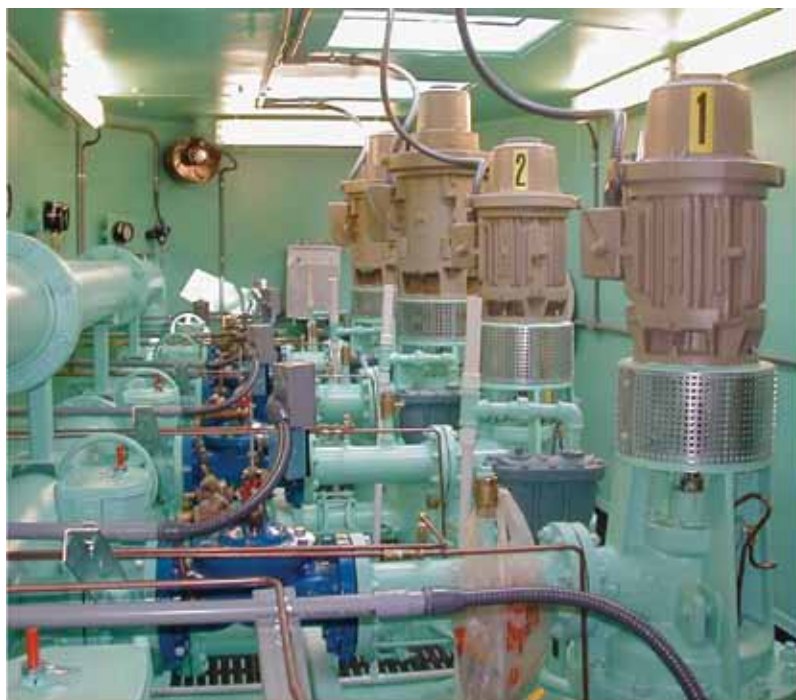
(Above) EFL factory built pump station, installed and operational in a fraction of the time it takes to build a pump station on site.
