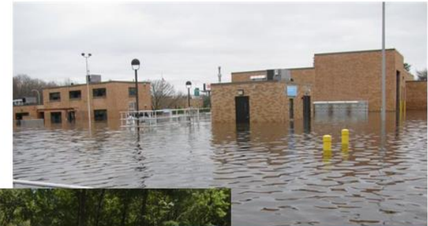
Warwick, RI WWTP, 2010 floods
