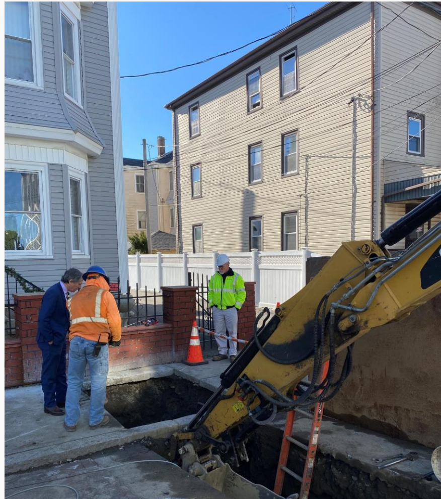
Lead Service Line Replacement (Fall River, MA)
